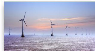
Renewable Energy / Electrification
